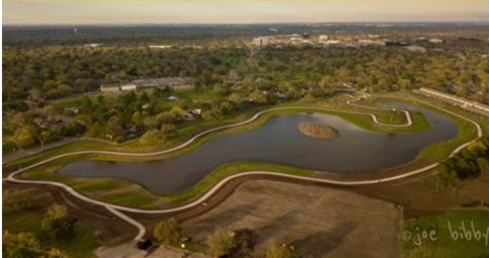
Figure 5: Aerial view of Phase 1
